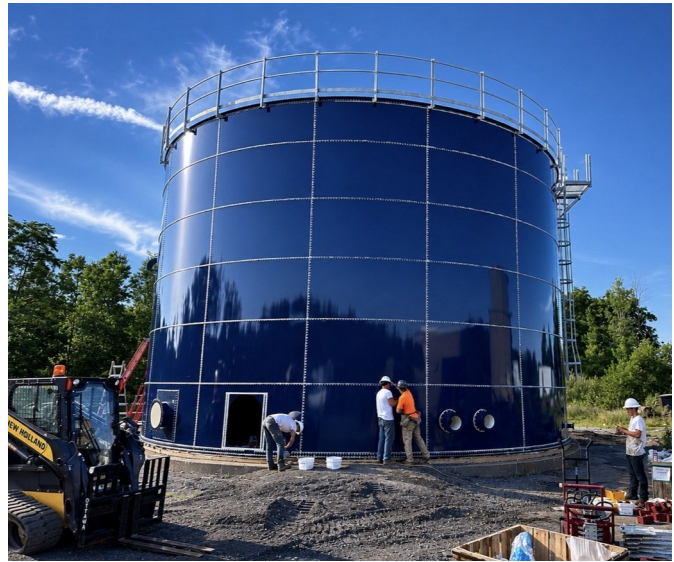
Photo 2 — The same tank complete: six rings of high-gloss FBE-coated sheets with staggered vertical seams, perimeter roof guardrail, caged ladder with step-off platform, shell manway and factory-located nozzles, awaiting the door-sheet closure and final sealant work at the base.
