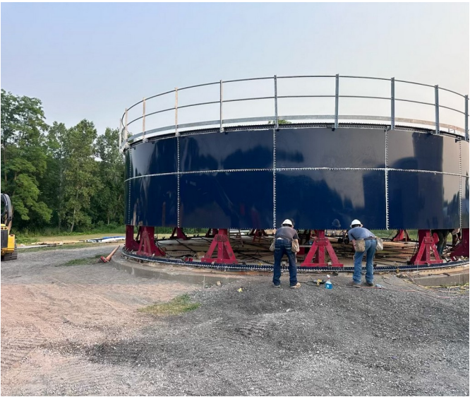
Photo 1 — Factory-coated (FBE) bolted tank under erection by the jacking method: the roof, guardrail and upper rings are assembled at grade and raised on synchronized hydraulic jacks, and each lower ring is bolted in beneath them — the crew never leaves the ground.
