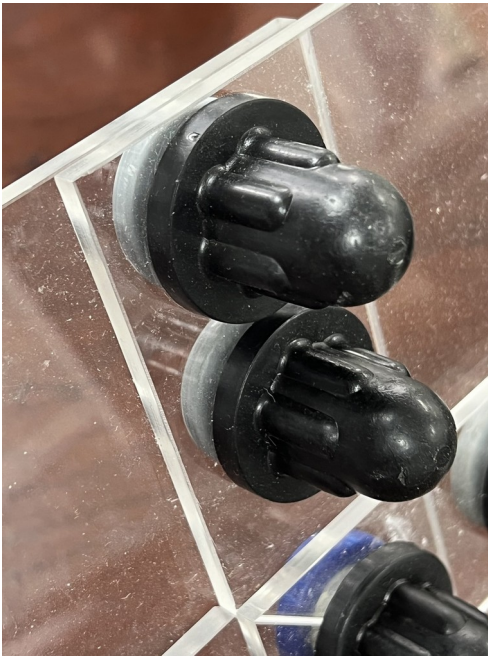
Photo 5 — Interior (wet) side: fin-neck bolt heads fully encapsulated in black UV-stabilized polypropylene up to the splines, so no fastener steel touches the water. In the typical potable design (Detail 4) the head is inside the tank.
