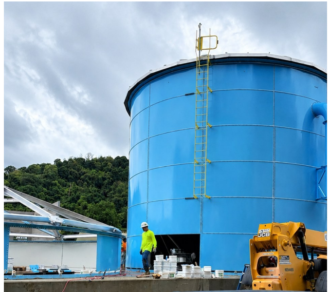
Photo 8 — Fusion-bonded-epoxy (FBE) coated tank nearing completion: exterior ladder with safety gate, external overflow downcomer, door sheet out at the base, and the bolted floor of a second tank being assembled on its slab at left.
